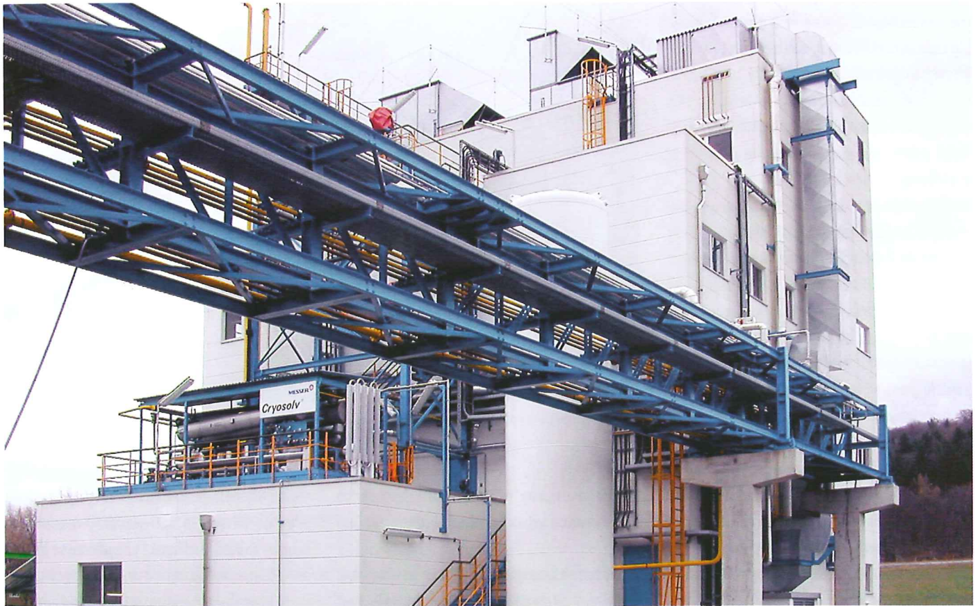
Figure 1: The new Chemetall Lithium-alanate production plant at Langelsheim/Harz is mainly classified as Zone 1 hazardous areas
