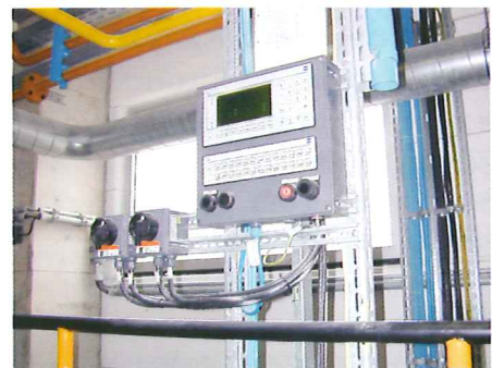
Figure 2: SAE-STAH displays as a local panel. These enable in-field intervention in specific production stages
