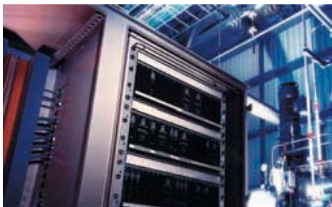
Figure 2: ICS MUX - Remote I/O, dating from 1990
